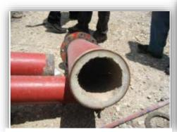
The pipeline to the power station was coated with a thick layer of extremely hard scale. Hydroflow prevented new scale from forming and began to remove existing scale.
