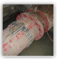
The same installation in 2010. No damage to the HydroFlow despite periods of submersion.
